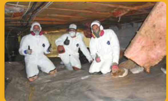
Contractors during a crawl space conversion.
